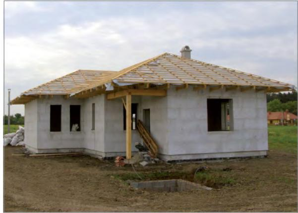
In ideal circumstances the building structure of a house with a floor space of 100-120 m<sup>2</sup> is finished within 16 days. During the on-site assembly the engineering works can be commenced, so this technology reduces the time necessary for the construction works of the building.
